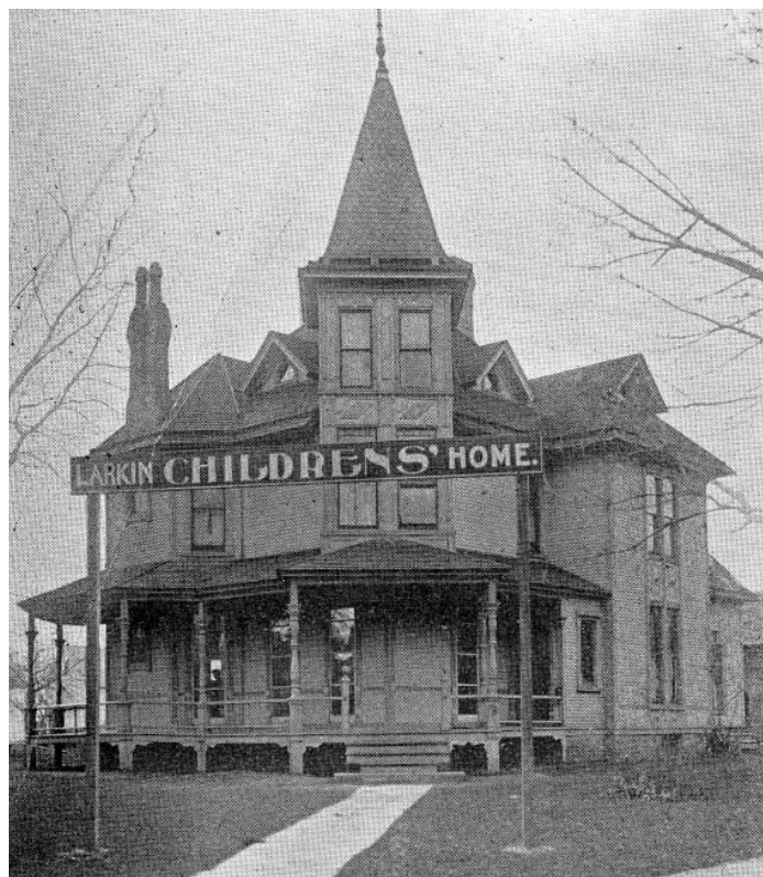
The Larkin Home at 352 South State St.
