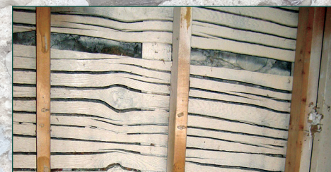
Interior, lathe for plaster wall peeled from a single log
