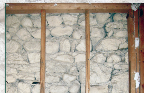
Interior, example of rubble walls 16" thick
