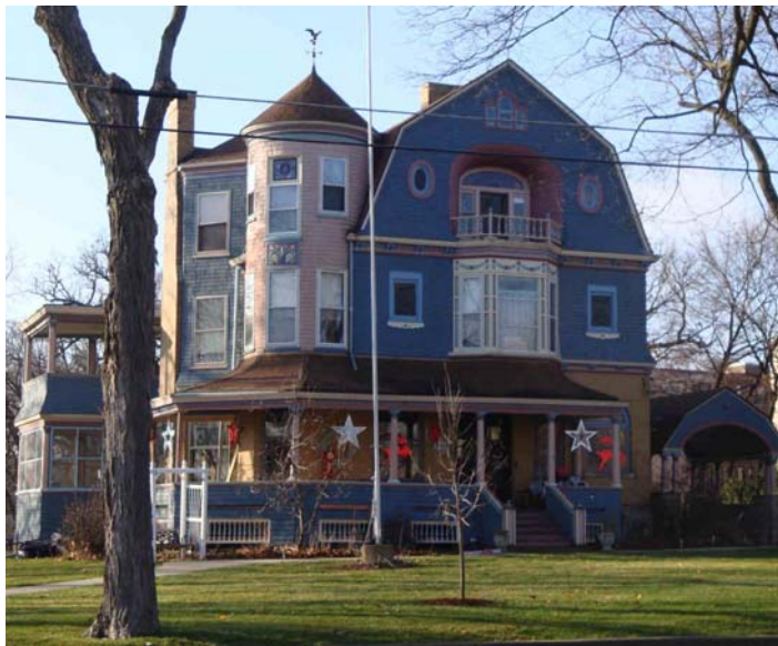
Jensen-built Queen Anne-style home, 705 W. Highland Ave
