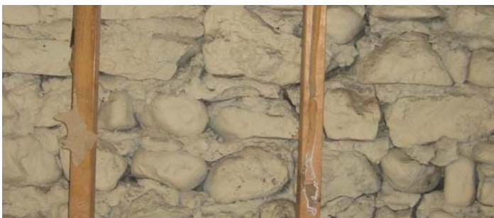
Inside of stone walls, showing rough fieldstone
