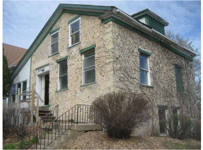
Kimball House, 302 W. Chicago St, from the southeast
