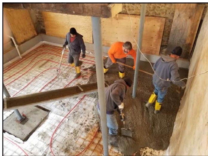
New concrete floor with radiant heating tubing
