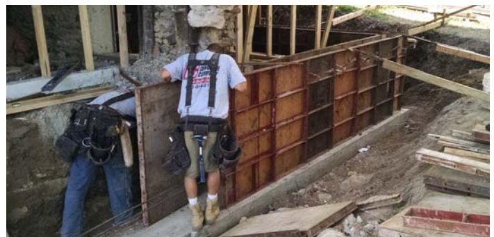
Putting up forms for pouring new concrete foundation
