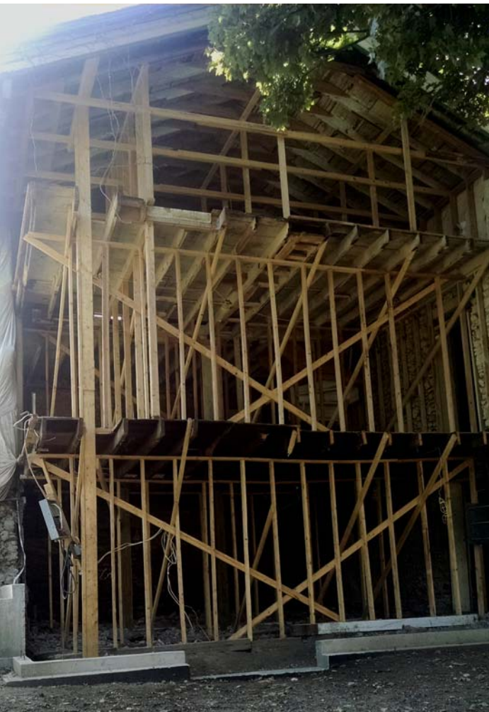
Back (north) wall completely removed and structure braced prior to rebuilding
