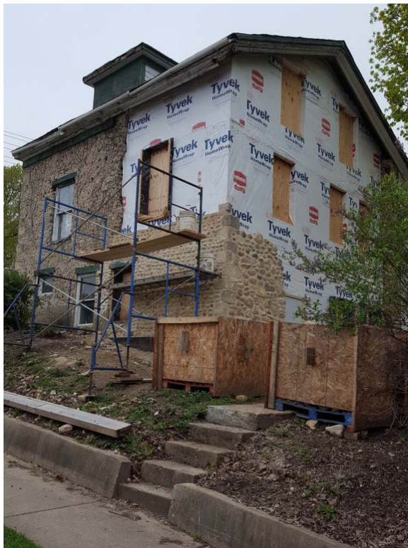
North and east walls of Cobblestone House showing cobblestone rebuild underway.
