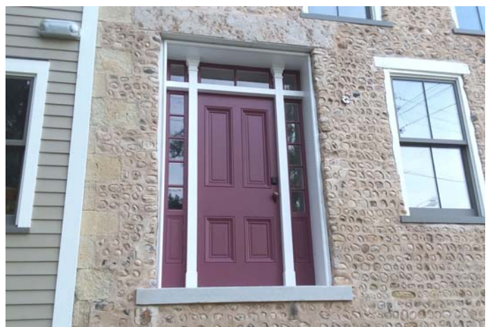
New front door, installed.
