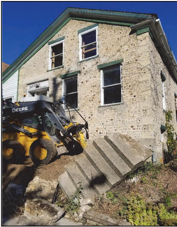
*Removing inappropriate concrete steps, 2017*
