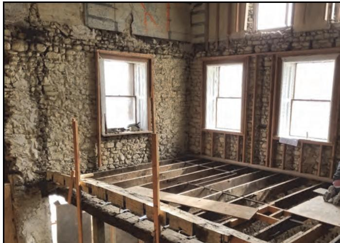
Gutted interior revealed cobblestone construction from the inside. Original beams were reused when possible. Photo from 2018.
